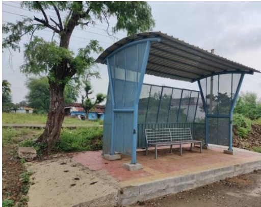
RR Constructions-Talegaon Project
